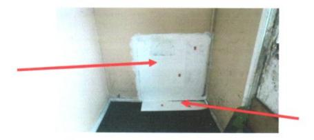
PLEASE REFER TO – SAMPLE No (3) - AMOSITE (BROWN) ASBESTOS FIBRES WERE NOTED WITHIN THE WALL & FLOOR PANELS WITHIN THIS AREA
