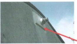
PLEASE REFER TO – SAMPLE No (4) - AMOSITE (BROWN) ASBESTOS FIBRES WERE NOTED WITHIN THE WALL & FLUE PANELS WITHIN THIS EXTERNAL AREA
